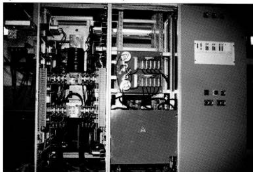
Figure 7: A TWIN POWER for 4.8 MW / 24-pulse
